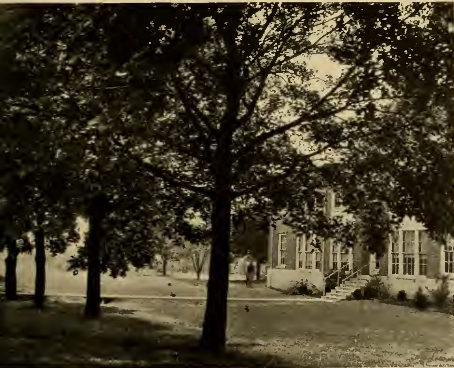
GIBBLE MEMORIAL SCIENCE BUILDING
